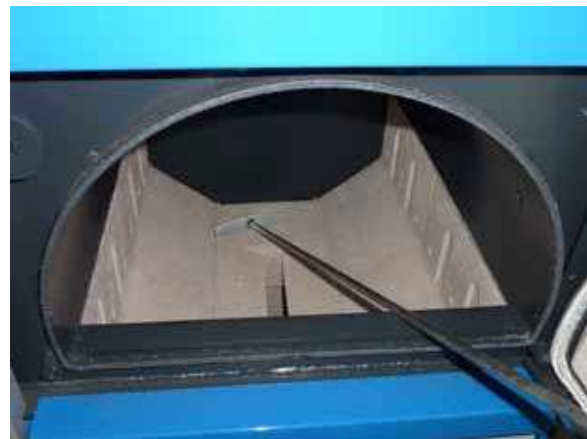
Sweeping the ash throught the nozzle down into the bottom (cleaning) chamber. The opening in the nozzle must be always clean and free.
